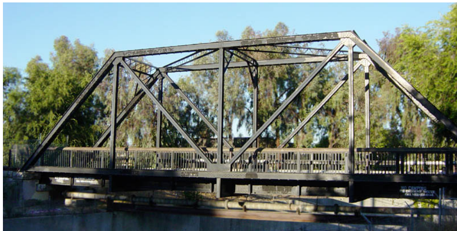
Figure 29 A simple truss
