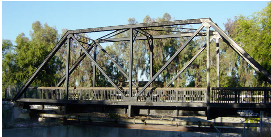
Figure 63 A simple truss
